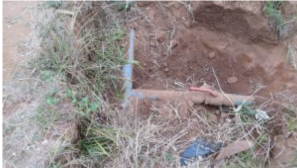
Gate valve regulating water to the 4 tanks from pan 1
