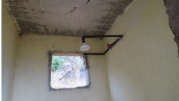
completed Showerhead of watchmen tower
