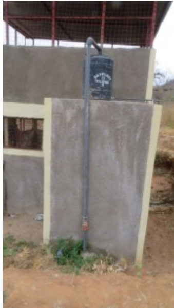
complete connection of pipe to the watchmen tower for the shower
